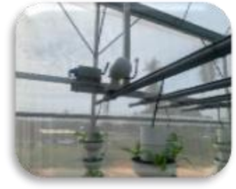
Indoor monitoring sensors
